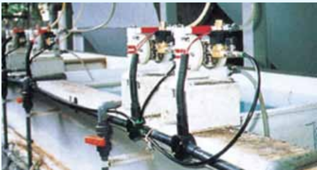
Blagdon 06 moulded pumps being used by Duraco Industries, Singapore, for chemical injection at a waste treatment plant.
