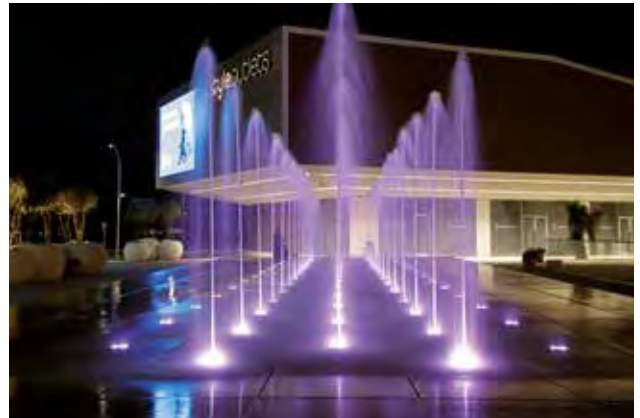
Style Outlets Viladecans – Barcelona, Spain
