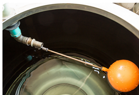
Level control float switch
